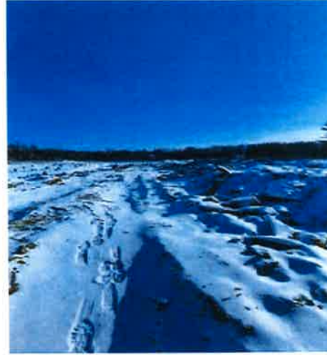
Photograph 2: Access Rd construction, SE beyond beaver dam.
