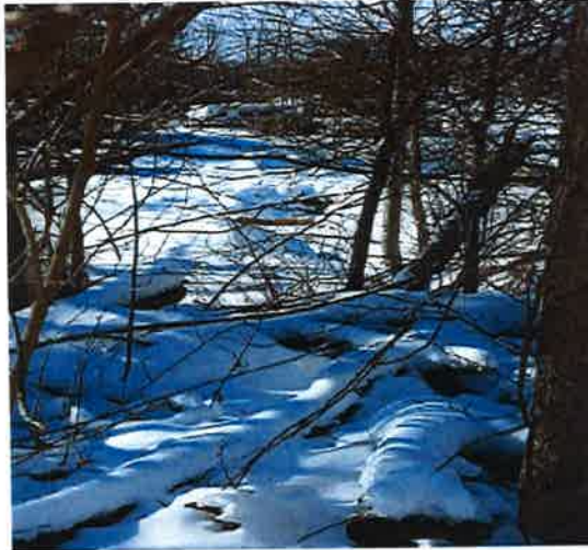
Photograph 5: Drainage swale, looking downstream (west) from 90 Swords Rd access lane. Straw bale check dam installed.
