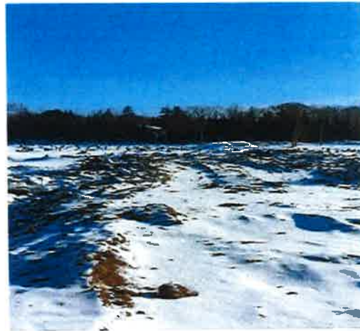
Photograph 4: Access Rd construction limits into beaver pond.
