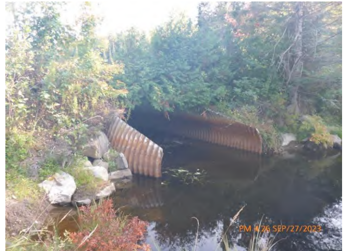
Figure 60 Poor Condition Culvert Example
