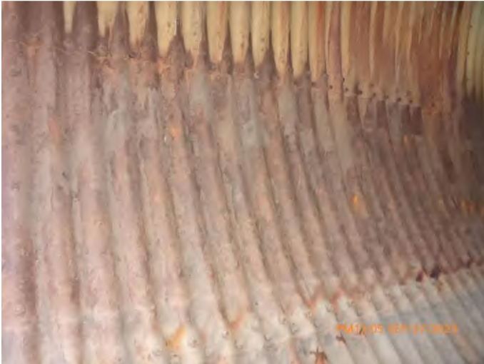
Figure 59 Fair Condition Culvert Example
