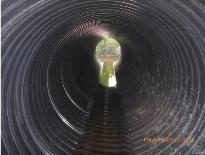
Figure 57 Good Condition Culvert Example 1
