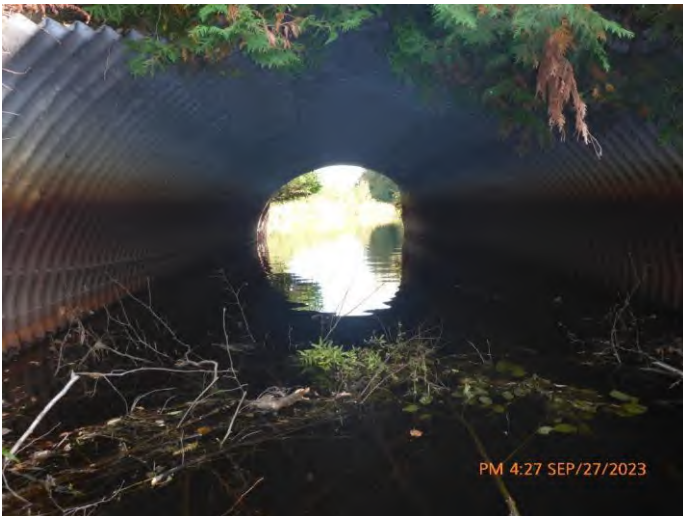
Figure 60 Poor Condition Culvert Example
