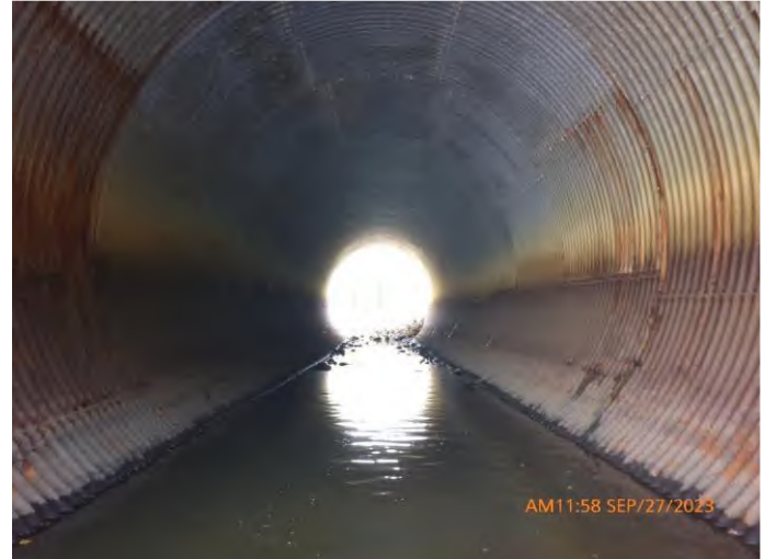
Figure 59 Fair Condition Culvert Example
