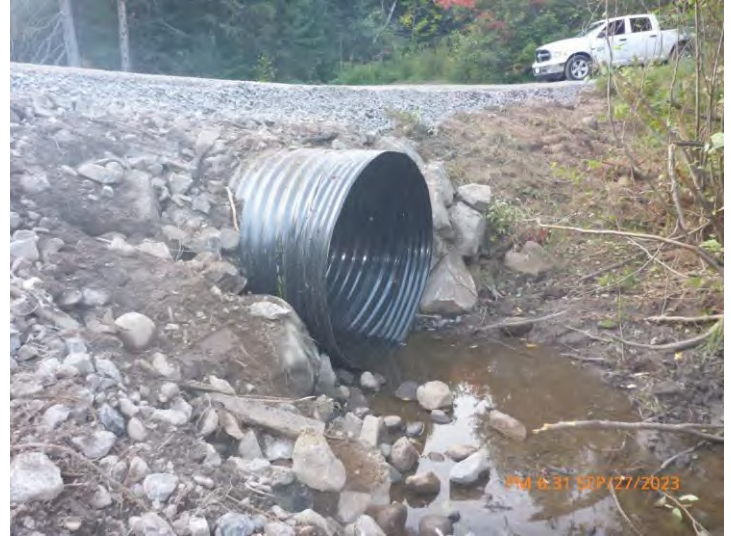
Figure 57 Good Condition Culvert Example 1
