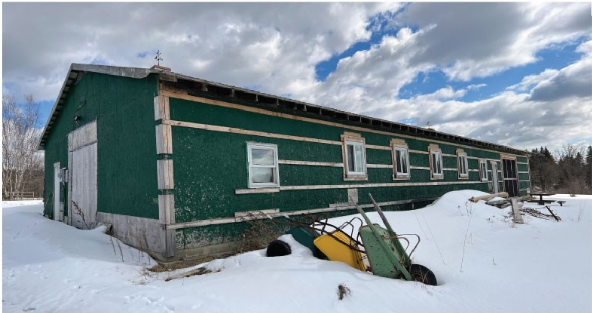
BARN ON RETAINED LOT
